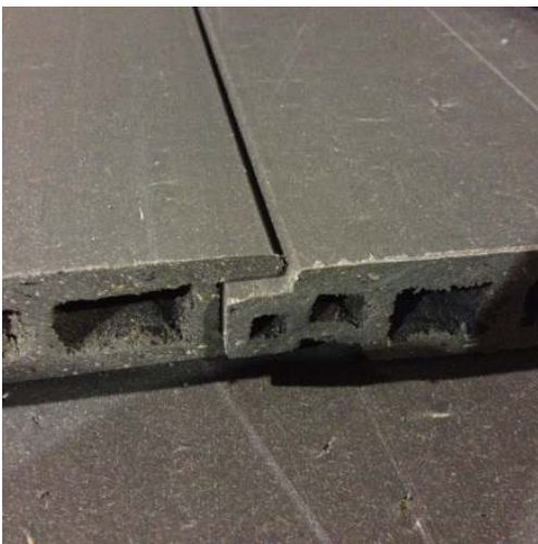
Tongue and groove joint
